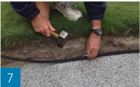
Optional drip-line irrigation installation on steep, dry faces. Drip-line irrigation is a US Patent a No. 13/822,799
