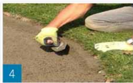
Optional forming of Capillary Bunker Edge
