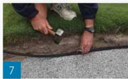
Optional drip-line irrigation installation on steep, dry faces. Drip-line irrigation is a US Patent a No. 13/822,799
