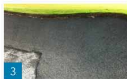
Spread Capillary Concrete at 2 inches (50mm) uniform thickness
